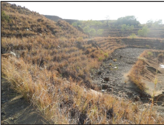
Figure 24. Vitiver grass used for slope stabilization is likely unstable and has limited economic value
