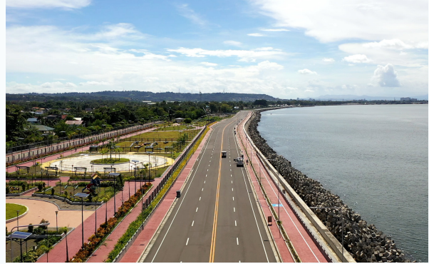
The Davao Coastal Road project aims to solve traffic woes in Davao and shall serve as a coastal shore protection and breakwater that will protect the city from sea waves and water surges.
